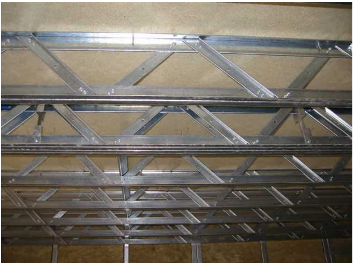
FIGURE 25 - LATTICE WEBBED "I" JOISTS
