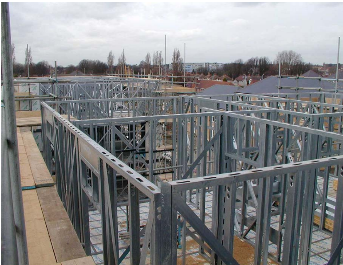
FIGURE 23 - STEEL FRAMES ASSEMBLED TOGETHER
